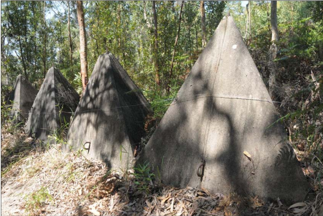
PLATE 3.3 View to northeast showing barbed and line wire linking tank traps in Lot 220
