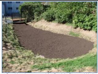
Macka's Bioretention Sand has been tested for Particle Size and Hydraulic Conductivity. The results are below. Macka's Bioretention Sand is a suitable sand component to any retention basin and can have up to 30% green waste added to create the whole profile necessary for filtering and managing water flow on sensitive sites. Product can be mixed at Macka's site upon request.
